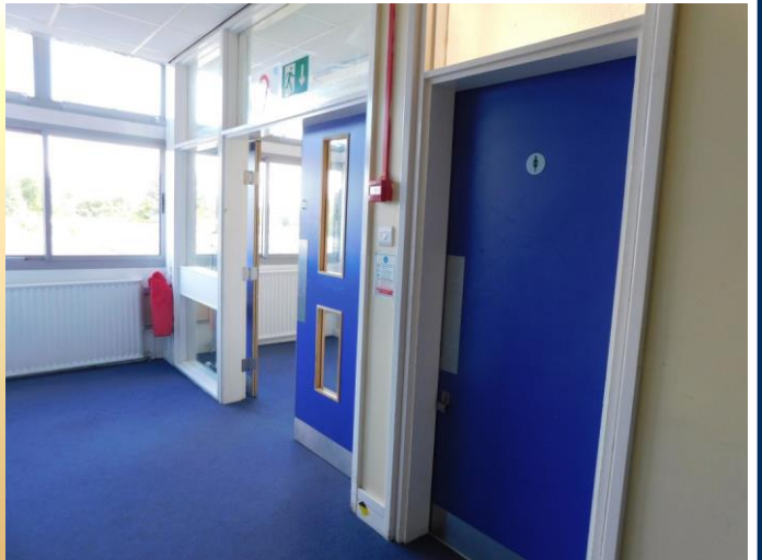
The Girls' toilets are on the top floor.
